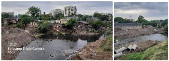
Ramnadi Stresses in Flood Plain: Cross section changed, Flood lines violated, Road Construction, Debris, Redundant old drainage lines
