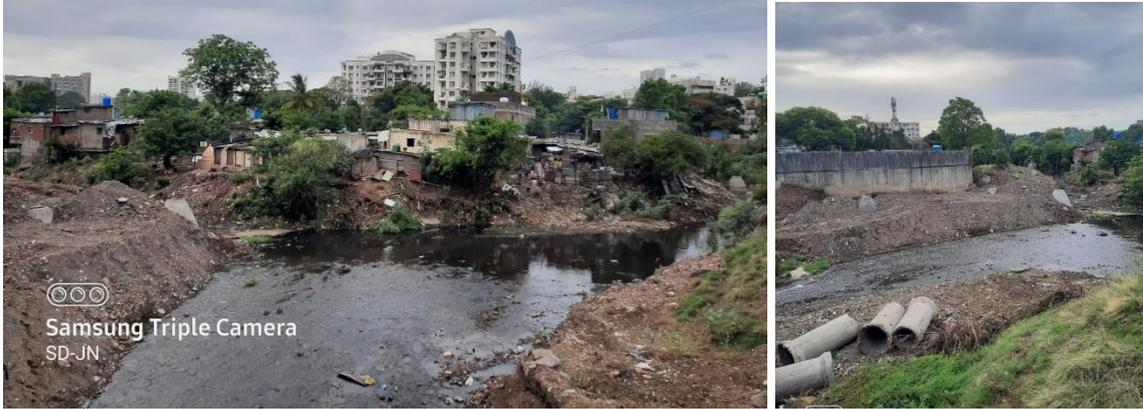
**Ramnadi Stresses in Flood Plain: Cross section changed, Flood lines violated, Road Construction, Debris, Redundant old drainage lines**
